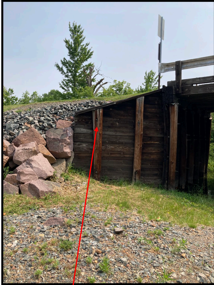
Deteriorating Wingwalls
